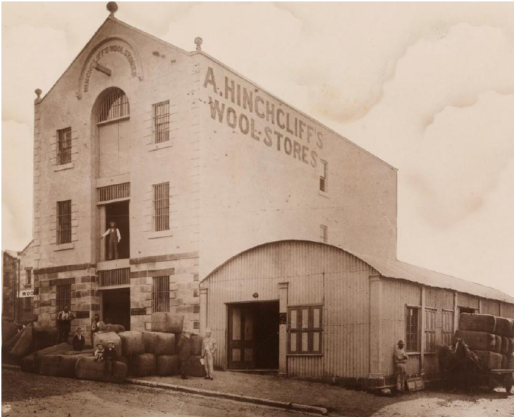
FIGURE 12 – HINCHCLIFF'S WOOL STORES, PRE-1882
